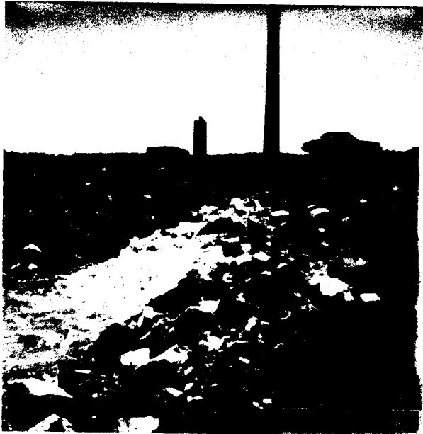
5 FLY ASH DISCHARGE CHANNEL.
