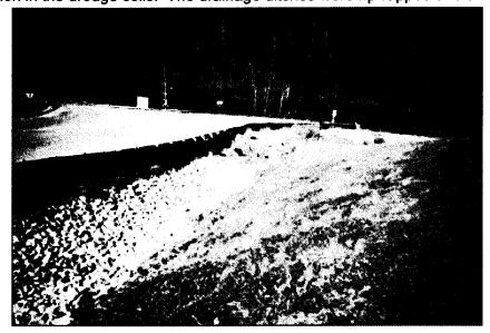
The intermediate soil cover was removed from the dikes between elevations 775 and 760 and stockpiled for reuse as a vegetative layer for cover. A non-woven geo-composite drainage layer was placed on the exposed ash and then recovered with one foot of soil.
