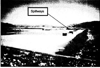
Sluice water flows from the active ash pond into the stilling pool through the five (5) new spillways constructed in 2005. The old plant constructed spillway (Kennedy Weir) were taken out of operation in 2005 as part a project to replace the Kennedy weir and allow more accurate accounting of free water volume. From the stilling pool, the water discharges into the plant intake channel via six standard spillways equipped with discharge diffusers constructed in November 2003.
