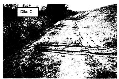
cover. The dikes had been mowed recently and were in very good condition. As shown to the left, some of the benches don't drain well. As much as practical, these ditches should be graded so they will drain, even if slowly. Wheel ruts that hold water should be filled with soil and covered with stone if they are in a road.
