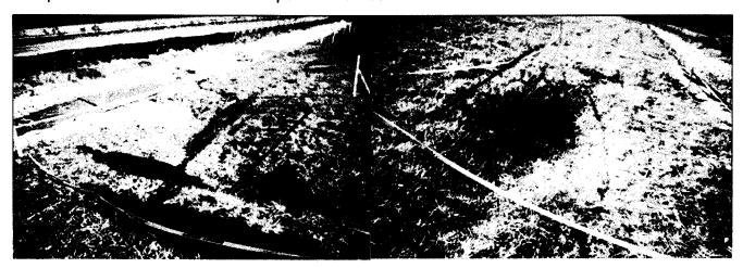
Since November 1, over 30 piezometers and a system of dewatering wells have been installed. The area has been excavated to investigate the cause of the failure. EDS and an outside consultant, Geosyntec, are working on a proposed solution, but as of this writing, a final recommendation has not been accepted.
