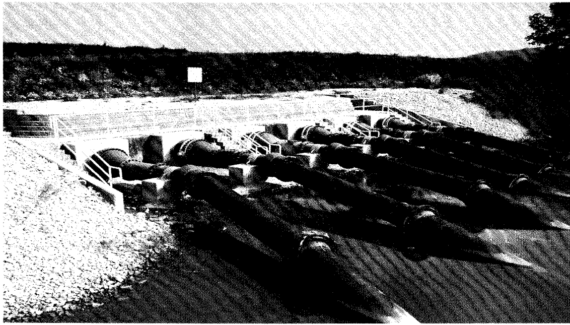
Picture 11: Discharge lines from stilling pond
