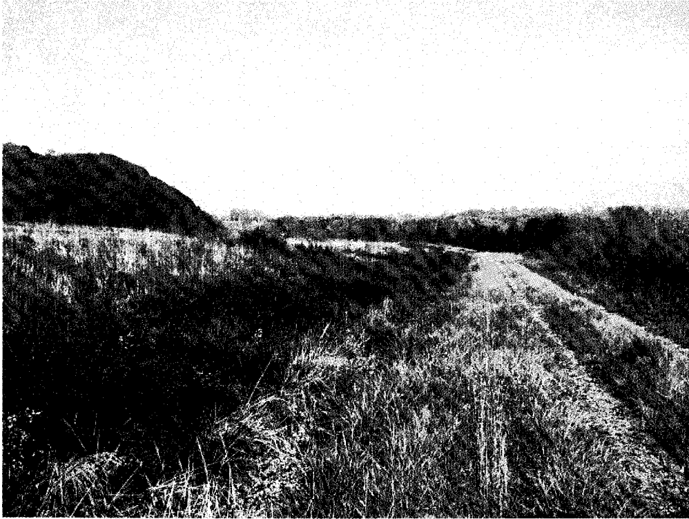
Photo 5—Looking northwest along Dike C roadway
