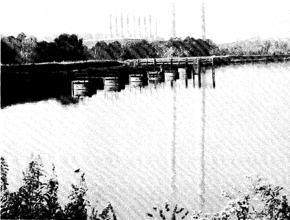
Photo 2—Looking southwest toward stilling pool spillways
