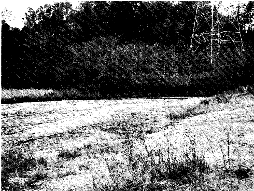
Photo 14—Looking southwest toward “wye” intersection with coal yard drainage basin
