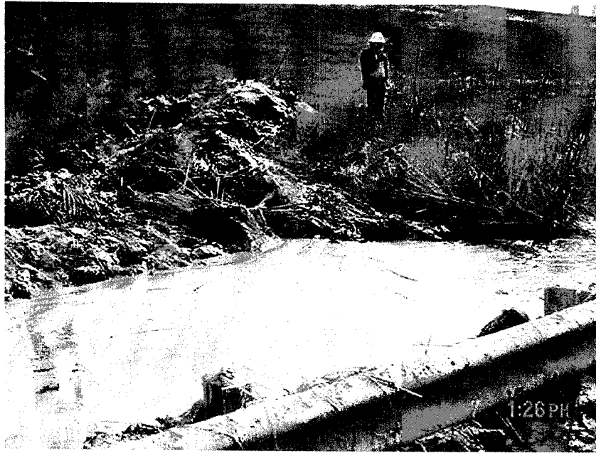
Photo 2. Leak in toe of the slope of dredge cell 2/3
