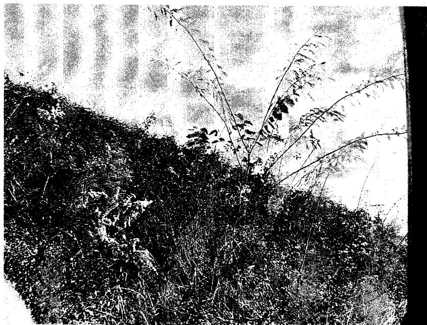
Photo 8. Heavy vegetation and small trees growing on the slope.
