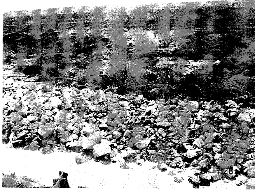
Photo 3. Ripraps put on toe of the slope to stabilize it.
