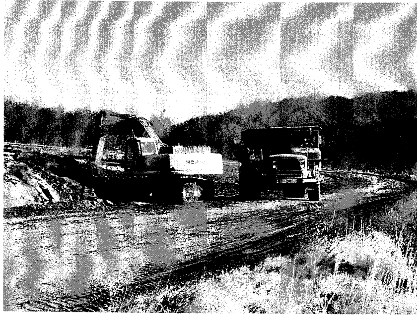
Photo 5 Ash is transported via truck to the top of Dredge Cell 1
