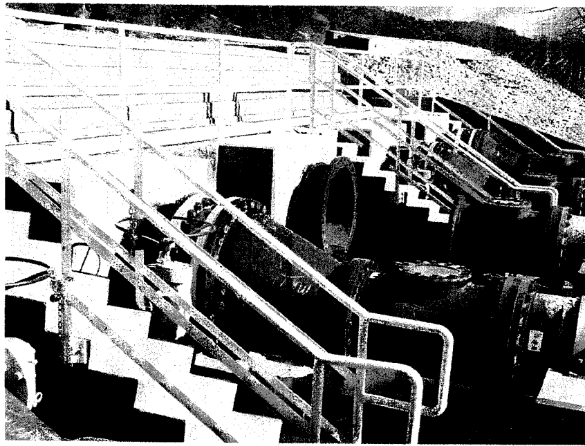
Picture 6. Ash Pond Discharge Diffusers
