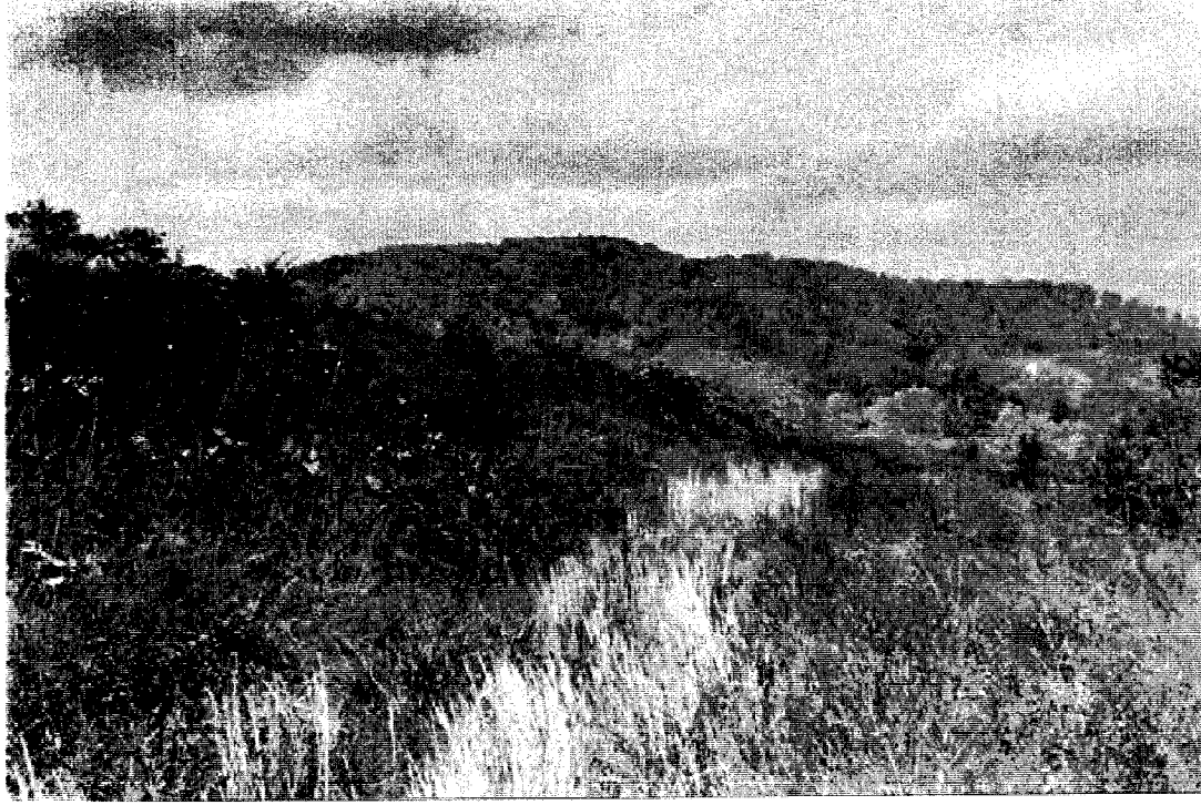
Photo 1 - Dike C and Lower Dike Road
