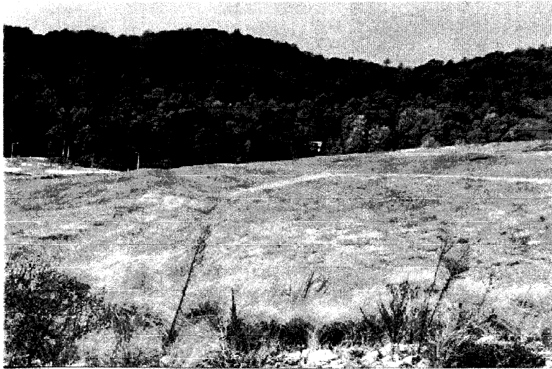
Photo 6 - Excellent Vegetation on Cell 1 Dike
