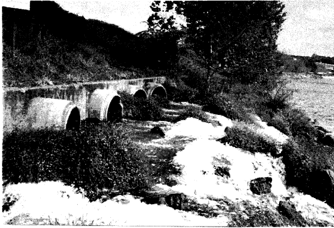
Photo 5 - Ash Pond Spillway Discharge
