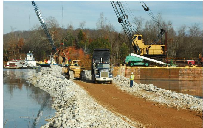
A second weir is being designed and when complete will confine the ash and keep it from entering the river during the river dredging process. This approximately 2000-foot rock weir will extend from Swan Pond Circle south to the plant river bank.
