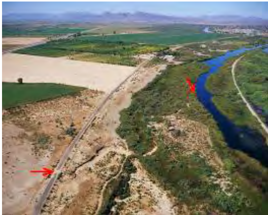
Figure 6. Red arrows show the beginning of the washout and its end at the backwater below the proposed CRIT 11 habitat creation site.
