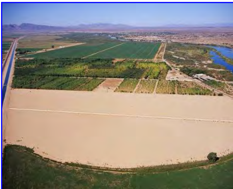
Figure 5. CRIT 10 cleared, and leveled with irrigation ditch midway across the site.
