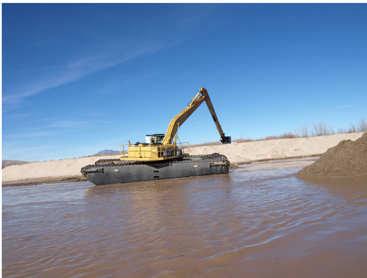
Photo 2: Amphibious excavator working on breach south of the Red Rock Staging Area (November 2010, Holste)
