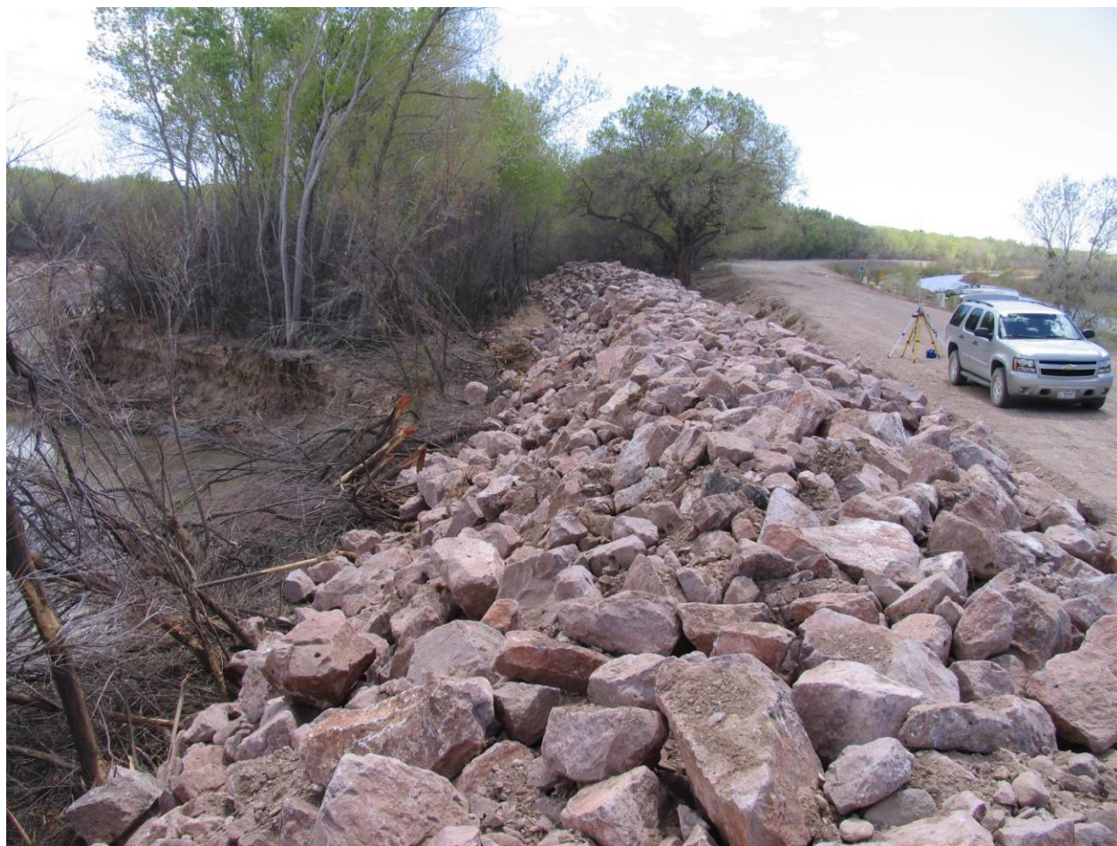
Photo 11: Fort Craig Bend riprap windrow, looking downstream (April 2011, Holste)
