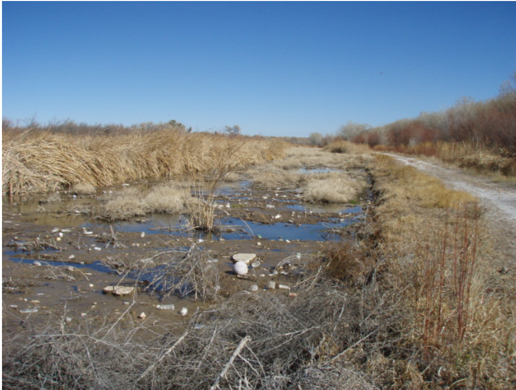
Photo 4: Tumbleweed plug within the LFCC (February 2011)
