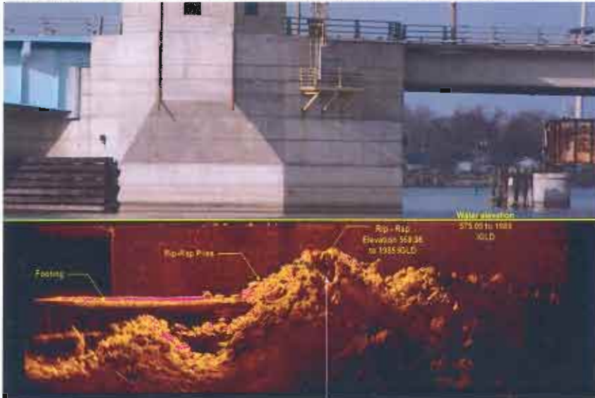
Vertical Visualization Upstream View of Pier Bullnose
