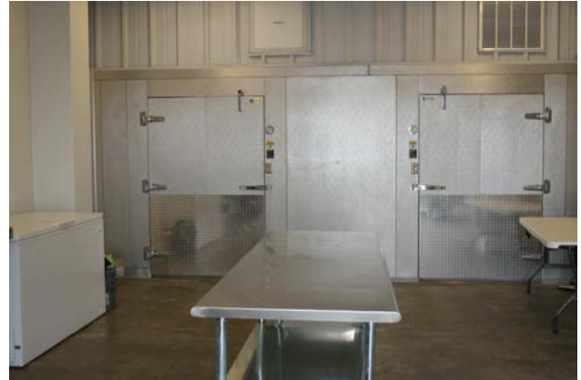
Inside of Necropsy Lab with freezer and cooler. Both are walk-in types capable of storing a large pilot whale carcass if necessary.
