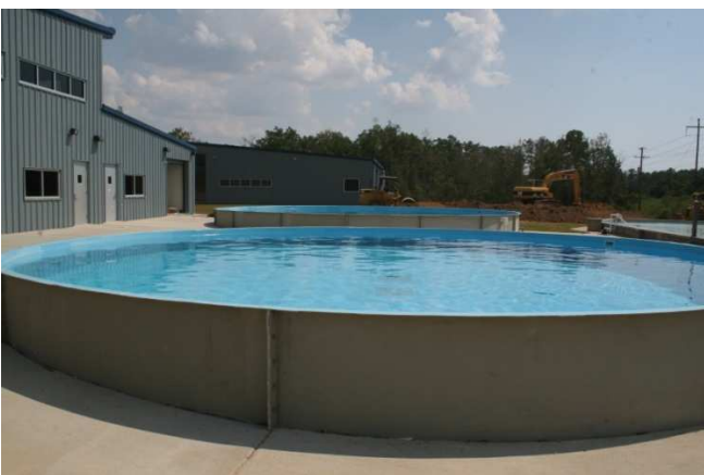
East view of dolphin rehab pools behind Animal Care building; 30-foot diameter pool is in foreground and 40-foot diameter pool is in background (30ft. pool is 8ft. deep and 40ft. pool is 10ft. deep).
