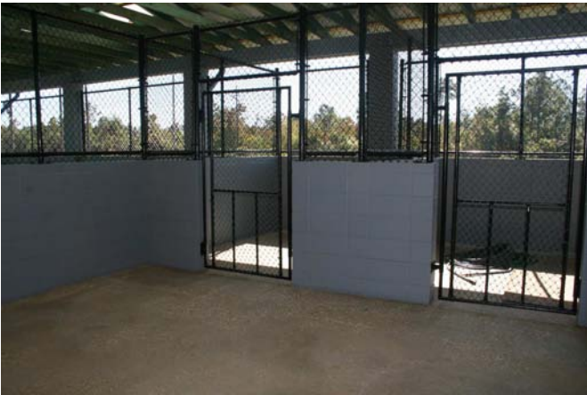
Interior holding pens.
