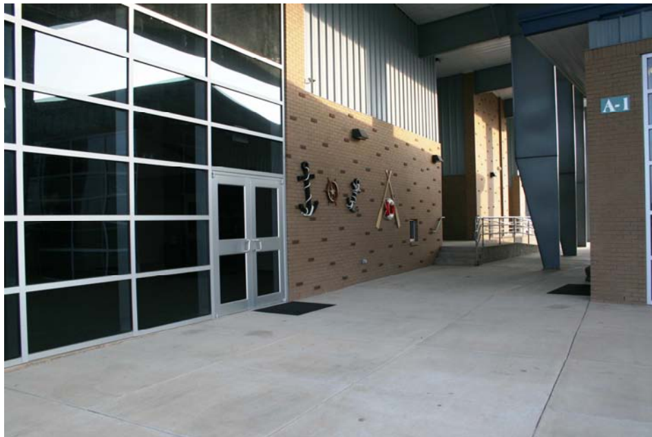
Breezeway and multimedia center.
