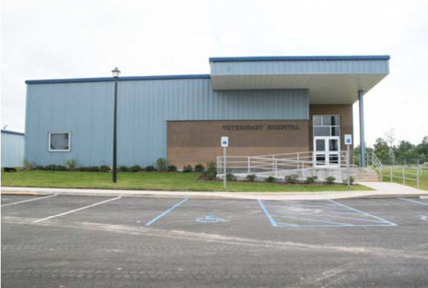
Front view (north side) of Veterinary Hospital.
