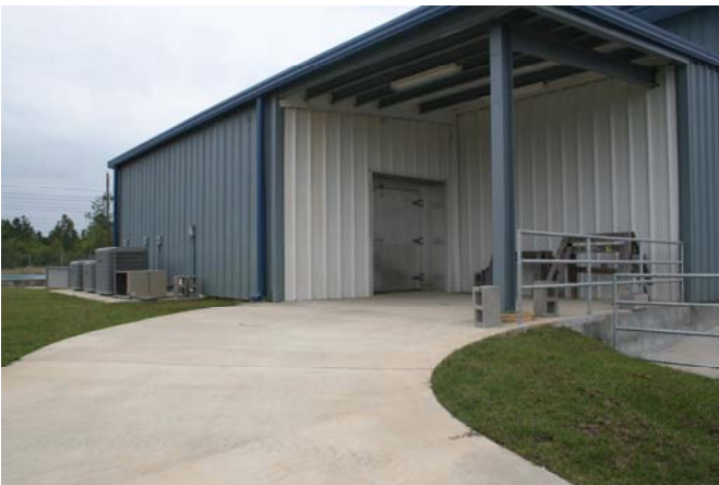
Close-up view of exterior entrance of fish freezer and ramp.
