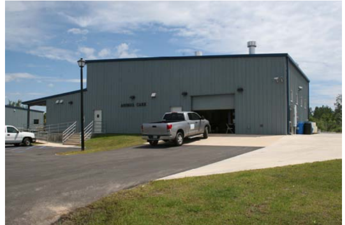
Another front view of Animal Care building.
