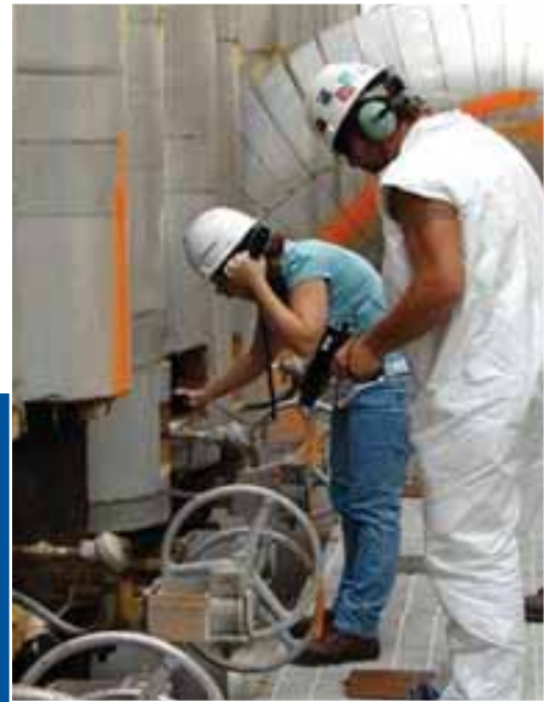
Technicians perform an ultrasound inspection of RC1 cooler piping.
