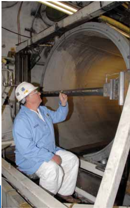
ATA Outside Machinist Jeffrey Fulmer conducts a test probe inspection at the APTU facility. The inspection was part of an ongoing major capability upgrade to APTU. The ongoing project includes a new combustion air heater (CAH) at APTU. The CAH, which underwent a successful preliminary burn using butane, is a crucial part of the upgrade, officially called the Hypersonic Air-Breathing Propulsion Test and Evaluation Capability. This upgrade has provided AEDC with a high fidelity flight simulation capability in support of emerging missile-class hypersonic weapon systems and vehicles.
