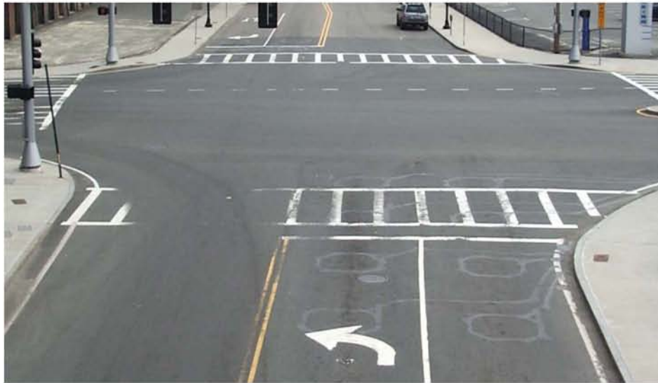
(b) Physical representation of loop detectors
