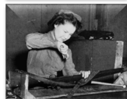
A WAC repairs a Springfield rifle at Camp Campbell, Kentucky
