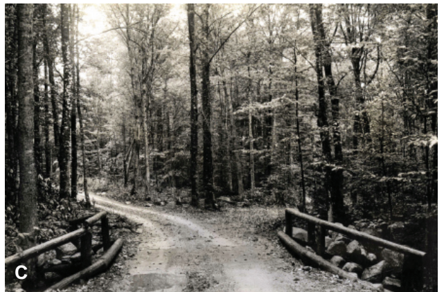
Figure 12.—The Bear Notch Road (A) was gravel until the 1950s; previously, it was the site of the Bartlett/Albany railroad track. The BEF interior roads (B) and bridges (C) were well developed by about 1934. U.S. Forest Service, Northern Research Station, Durham, NH.
