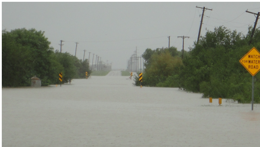
Record flooding on the Oso Creek in September 2010
