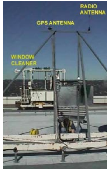
Figure 4. Deployed GPS unit and necessary frame system (Los Angeles, CA).
