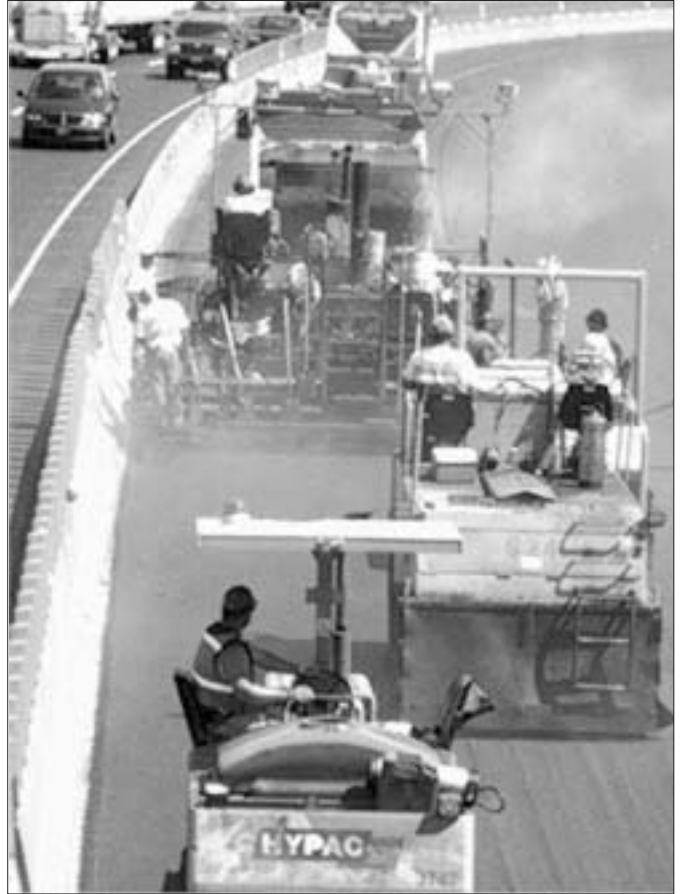
Figure 3 – Nearly 80 million pounds of asphalt were delivered in less than 100 hours
