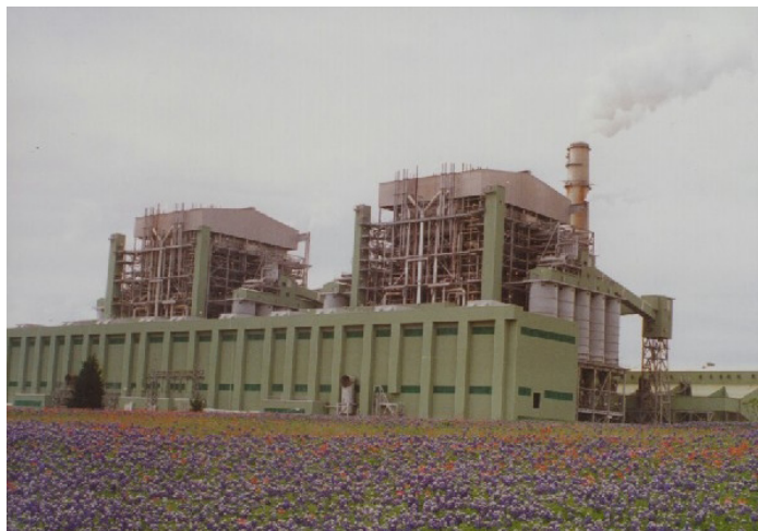
Texas Genco's Limestone Steam Generating Station
