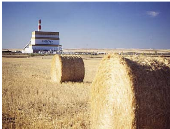
Poplar River Plant
