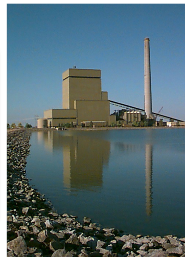
450 MW Big Stone Power Plant
