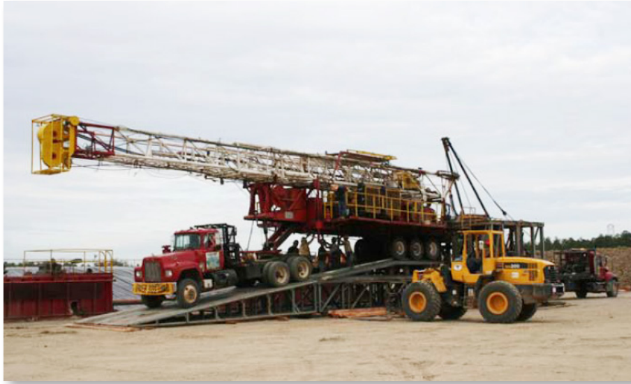
Drilling rig at Mississippi Test Site
