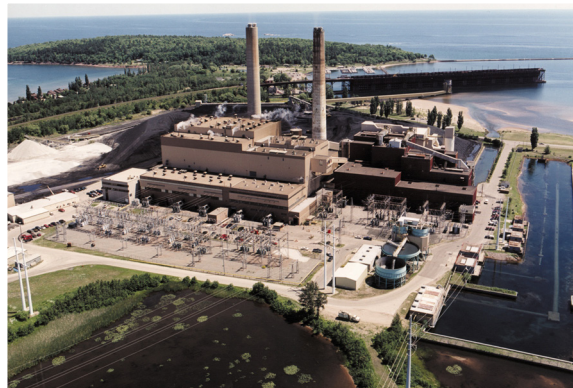
Presque Isle Power Plant
