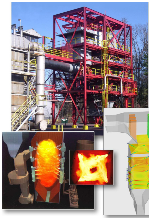
T-fired boiler design and boiler simulation
