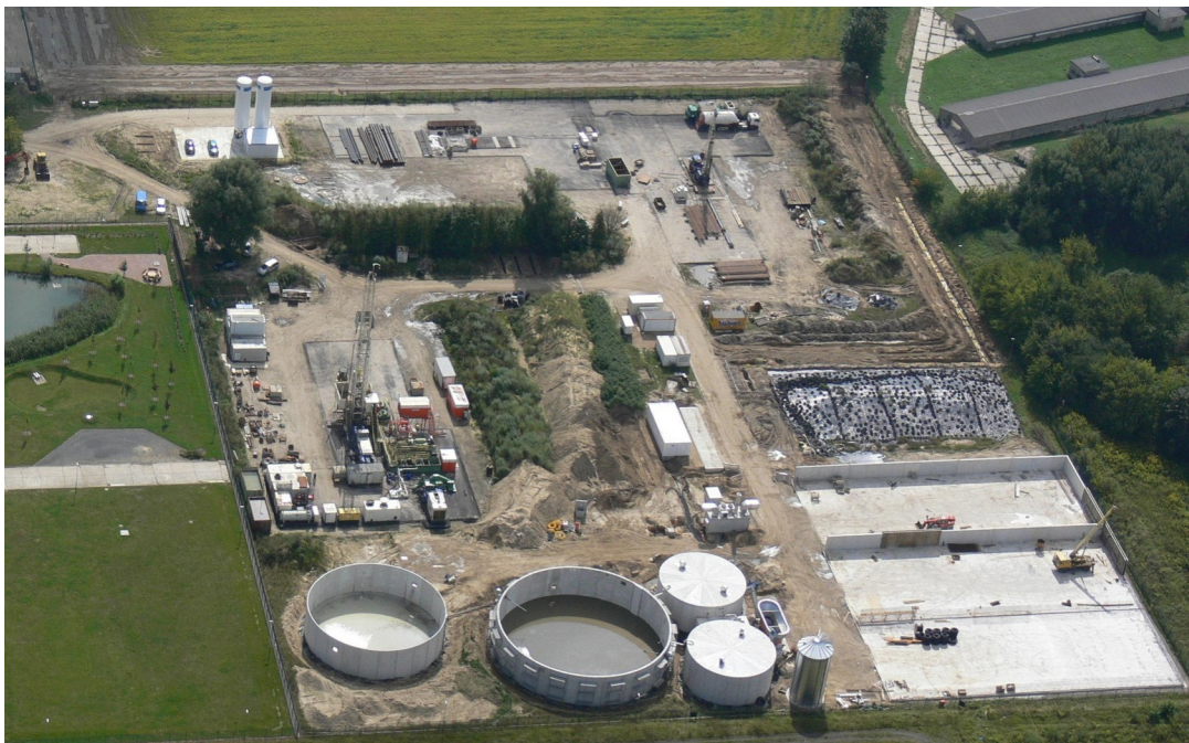
Figure 2: Aerial view of the CO 2 Storage Site (CO 2 SINK Project) in Ketzin, Germany. Picture is from www.co2sink.org .
