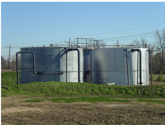
Figure 2: Water storage tanks storing produced formation water from an oilfield enhanced oil recovery (EOR) operation injecting CO 2 .
