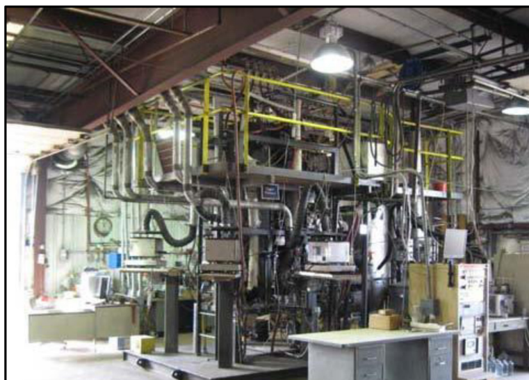
WRI coal combustion test facility.
