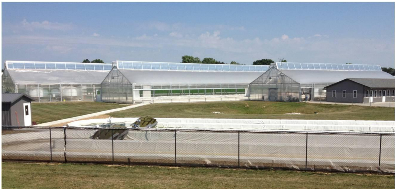
Touchstone Research Laboratory's Pilot Algal Facility at Cedar Lane Farms
