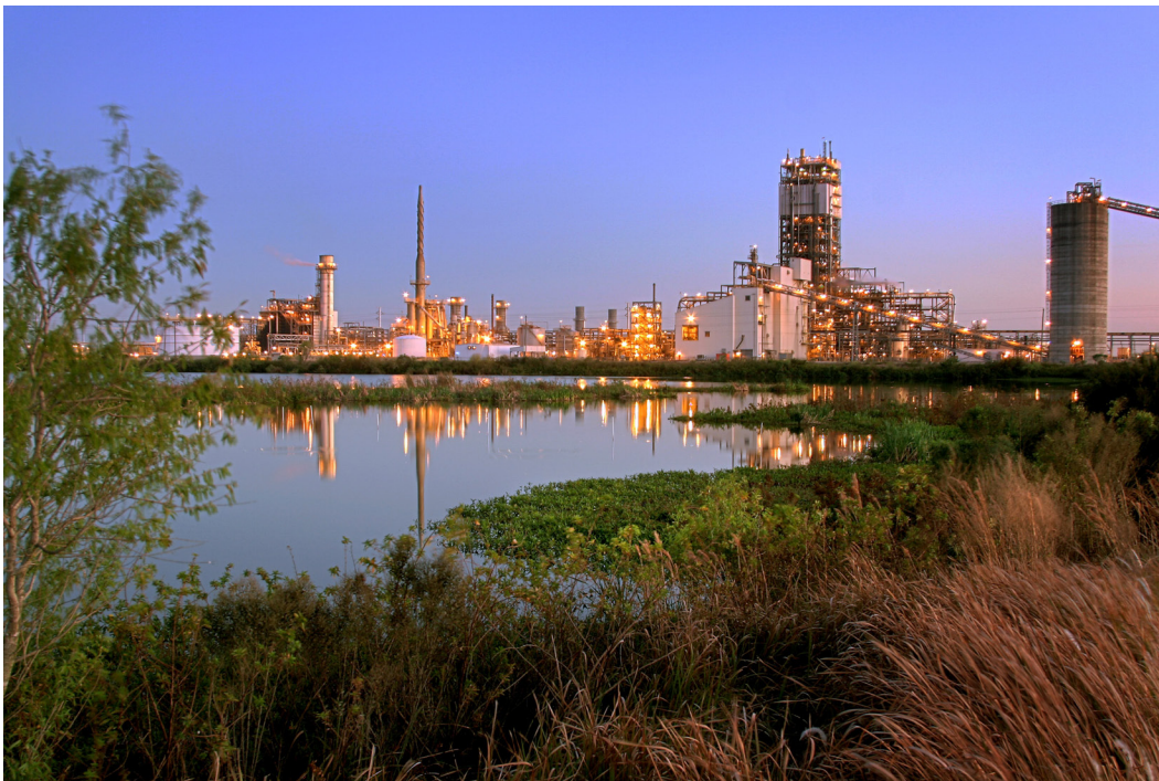
Tampa Electric Company's IGCC Plant, Polk Power Station
