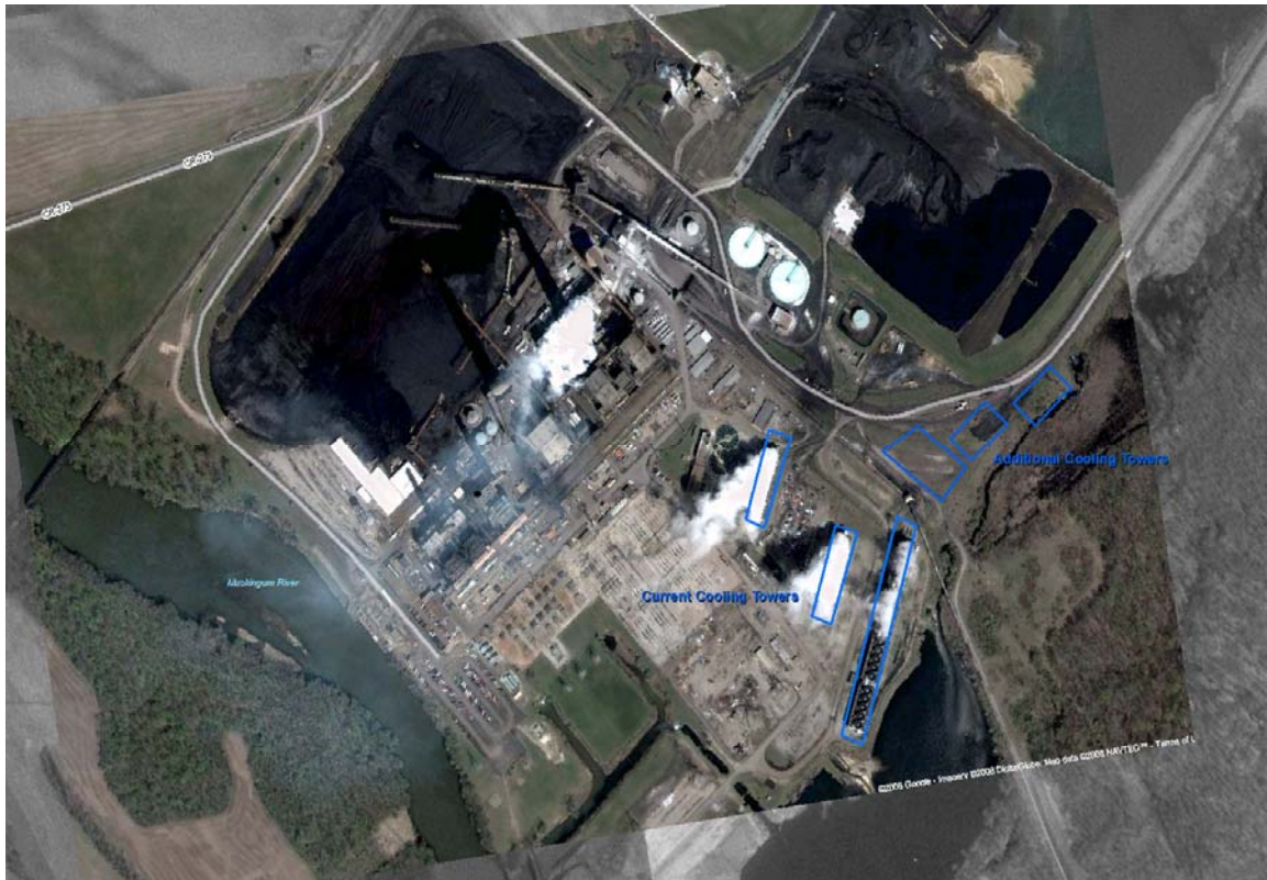
Figure 1-14. Current and Additional Recirculating Cooling Required to Retrofit All Units with 90% CO 2 Capture and Compression at the Conesville Plant
