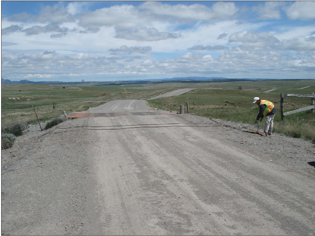
Site 009 Deadman Road Looking East
