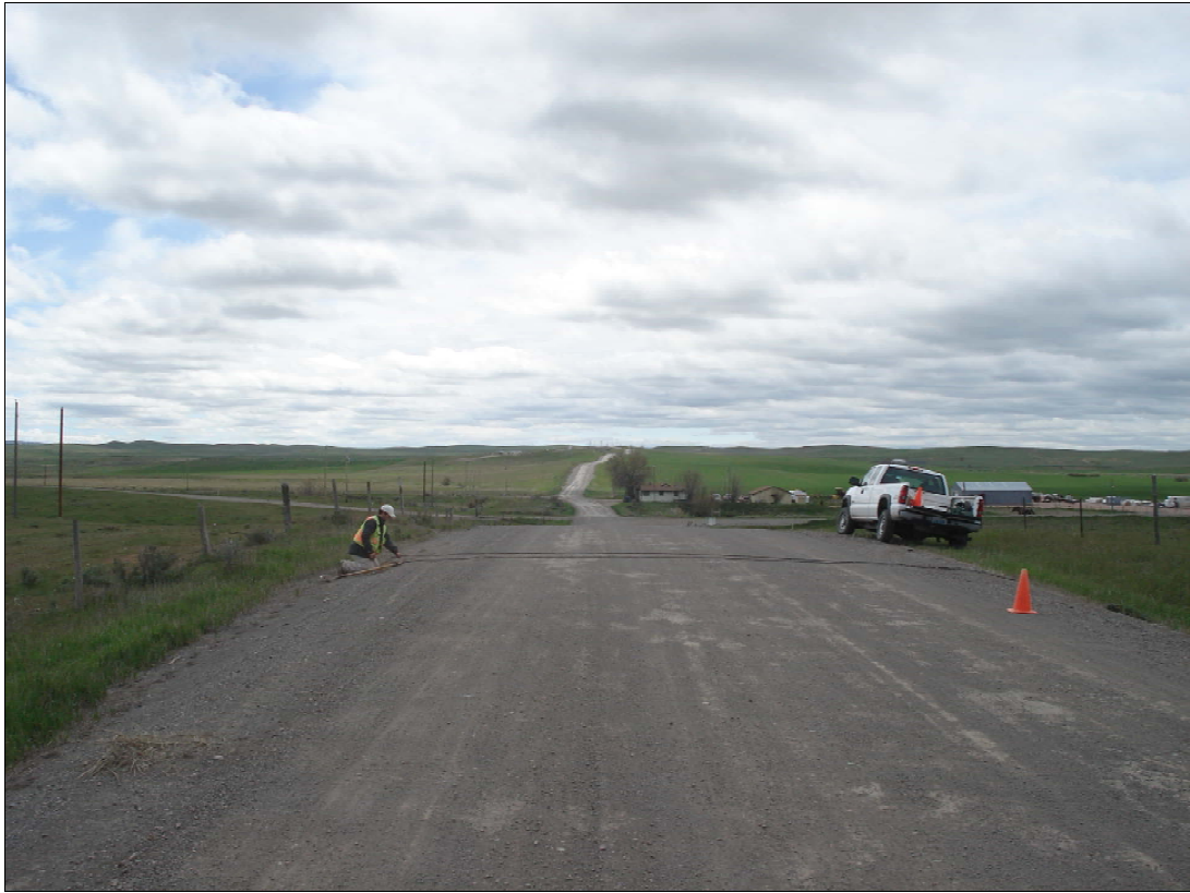
Site 005 New Haven Road Looking South
