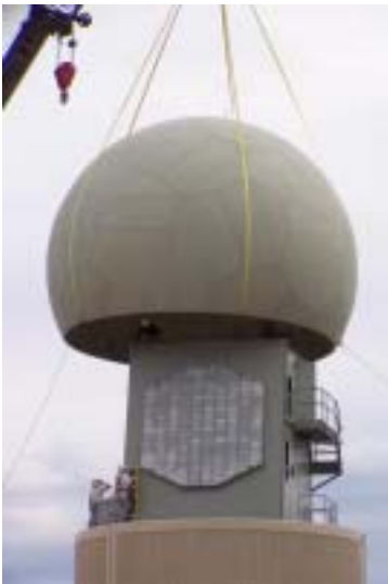
Installation of the dome
