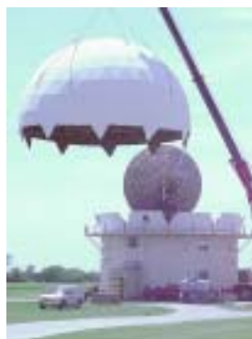
A crane lifts the radar dome off its base.
