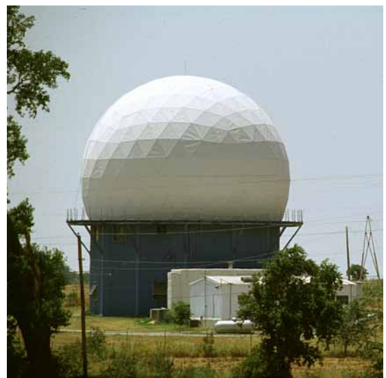
Figure 3: NSSL's Cimarron radar (CIM) will obtain measurements of polarimetric quantities along with reflectivity and Doppler velocities.
