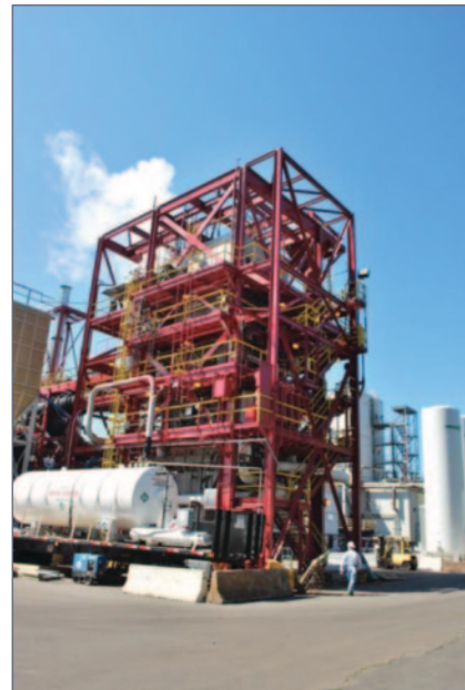
Figure 2: Alstom 15 MW th Boiler Simulation Facility
