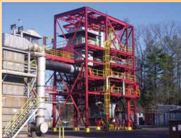
Alstom's Oxy-Combustion Test Facility
