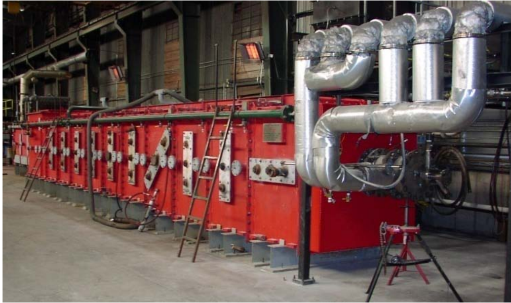
Figure 2: Pilot-Scale Combustion Facility (L1500)
