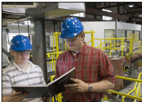
Figure 4: UNDEERC Post-Combustion CO 2 Capture Test Facility
