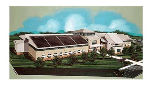
Aggressive passive solar orientation with east/west axis, roof overhangs, north and south facing windows and clerestories boost natural daylighting while reducing heating and cooling loads, reducing HVAC system cost, and optimizing year-round energy performance.
