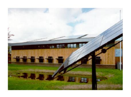
A truly integrated design approach and effective use of various "Green for Less" strategies and technologies enabled PA DEP to install a 14 KW PV array within the modest budget.
