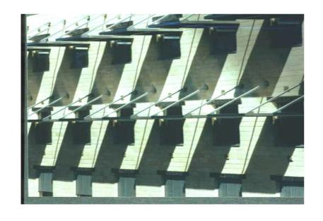
Exterior light shelves bounce daylight into the occupied spaces of the building improving indoor ambient lighting levels.
