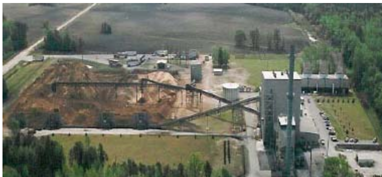
Photo of Craven County Wood Energy
