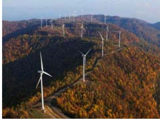
Buffalo Mountain, Tennessee: 15 Vestas 1.8 MW Wind Turbines.
