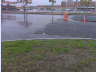
Pervious pavement installed by Maine DOT in partial support of Long Creek Watershed Management District (LCWMD)
