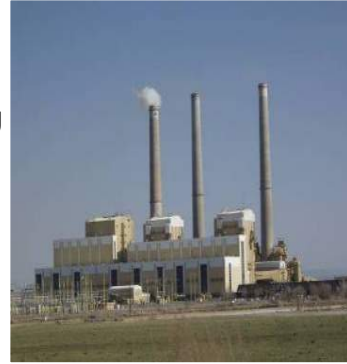
Coal-fired electric power plant
