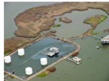
Source: Louisiana DEQ Flooded Wastewater Treatment Plant
