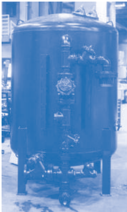
Figure 7-7. Pressurized Media Filter (USFilter).
