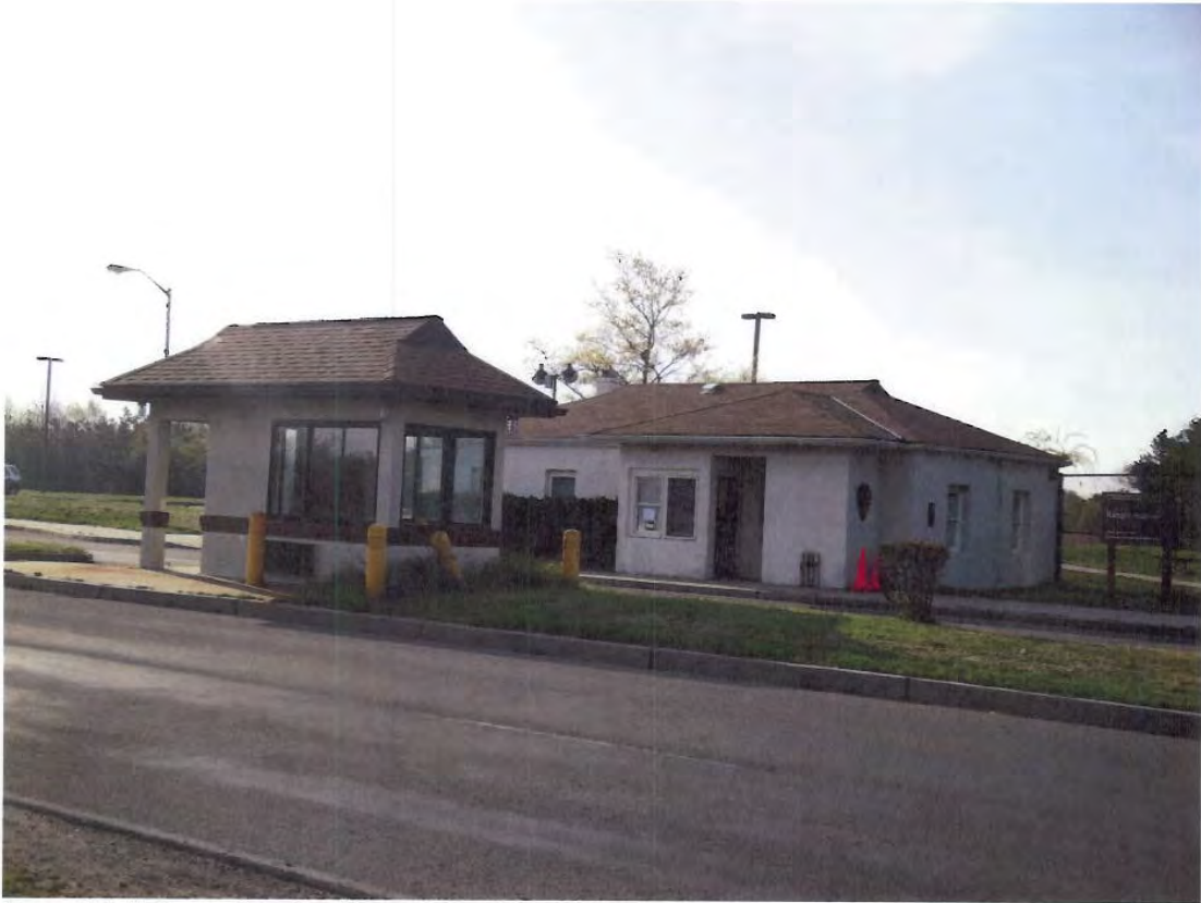
Figure 15: Entrance booth and Ranger Station at west entrance to Park. View to the south.
