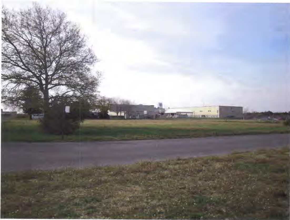
Figure 18: View of western portion of Officer's Quarters loop road with MARFORRES Center in background. View to south.
