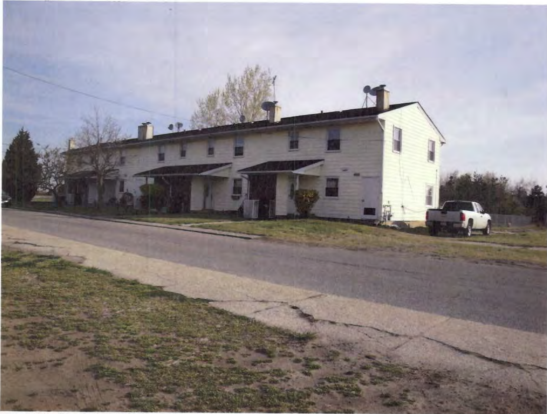
Figure 14: Married enlisted men's quarters (now Park staff housing) in west barracks area with Aviation Road in foreground. View to the east.
