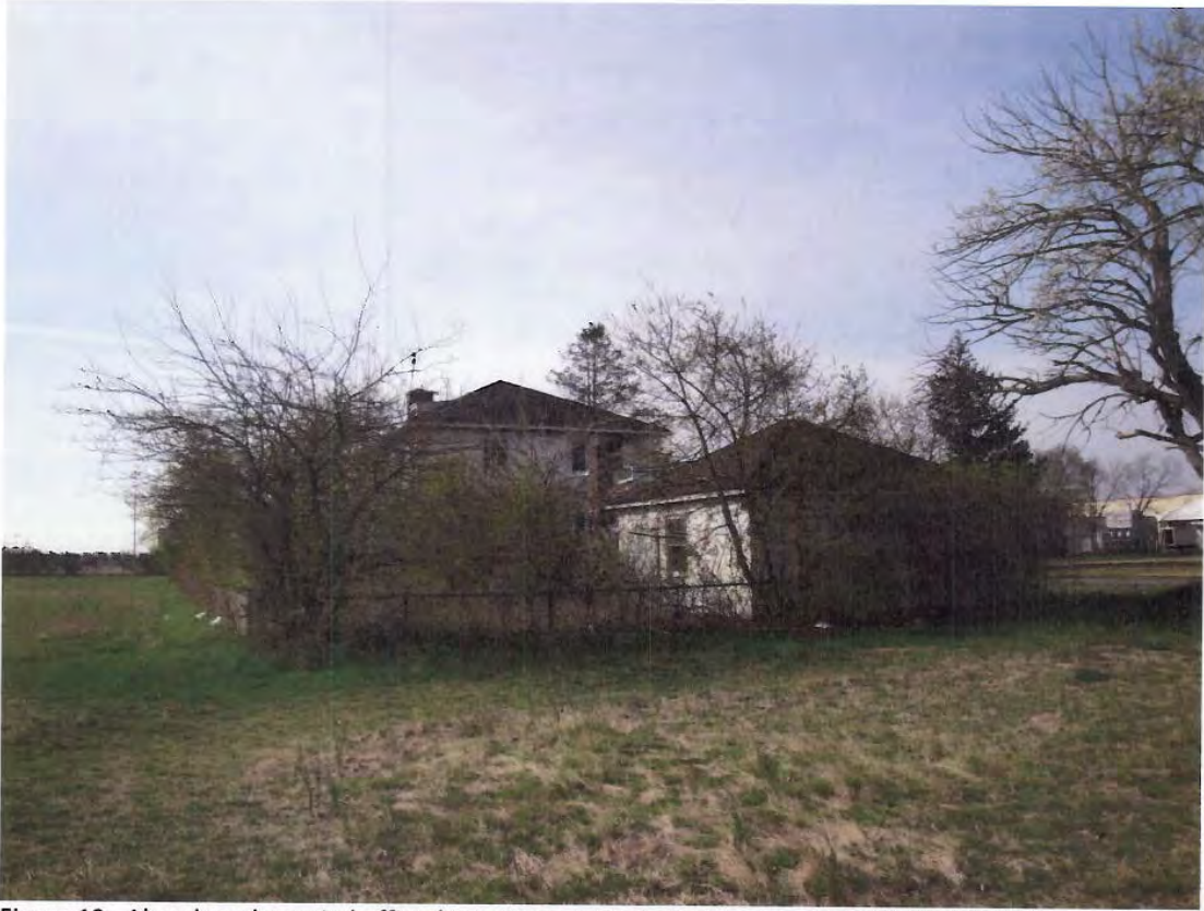
Figure 12: Abandoned married officer's quarters, main barracks area. Note MARFORRES Center in background at right. View to northeast.
