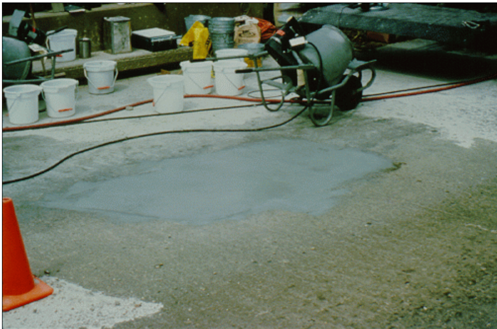
Figure 59.—Polymer concrete must be protected from water and not disturbed during the 1- to 2-hour curing period. No other curing procedures are required unless ambient temperatures are very low.
