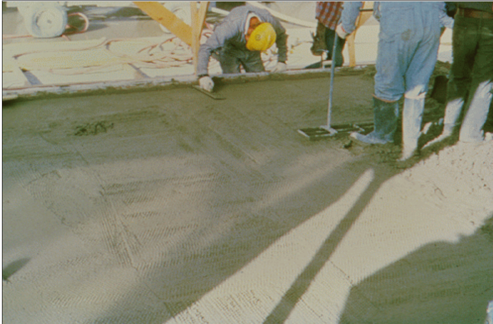
Figure 52.—Epoxy mortar is consolidated and compacted by hand tamping.
