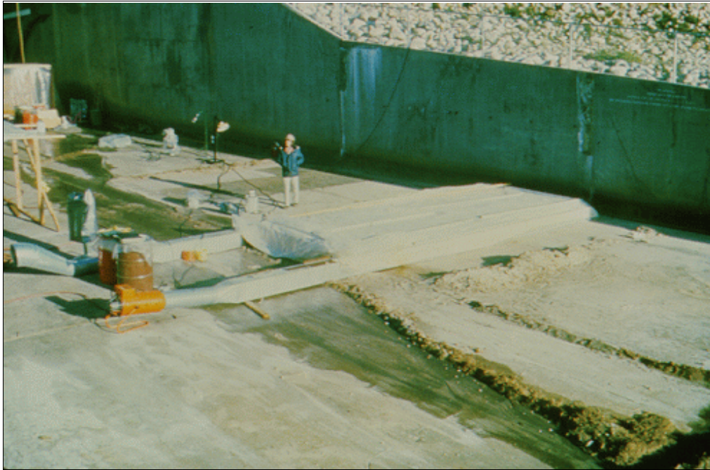
Figure 54.—Postcuring heating enclosure installed over an epoxy mortar repair area.
