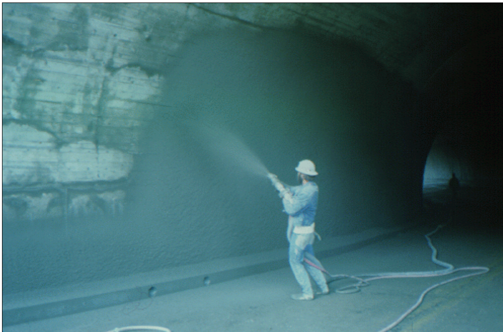
Figure 46.—Wet mix shotcrete is propelled by compressed air.
