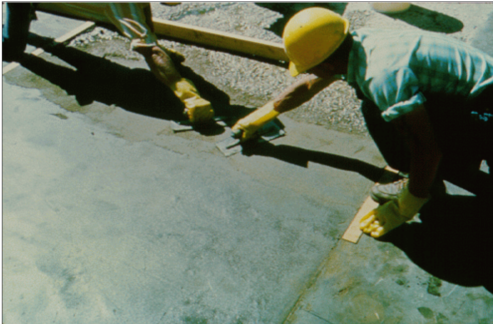
Figure 53.—Applying the steel trowel finish required by epoxy mortar repairs.
