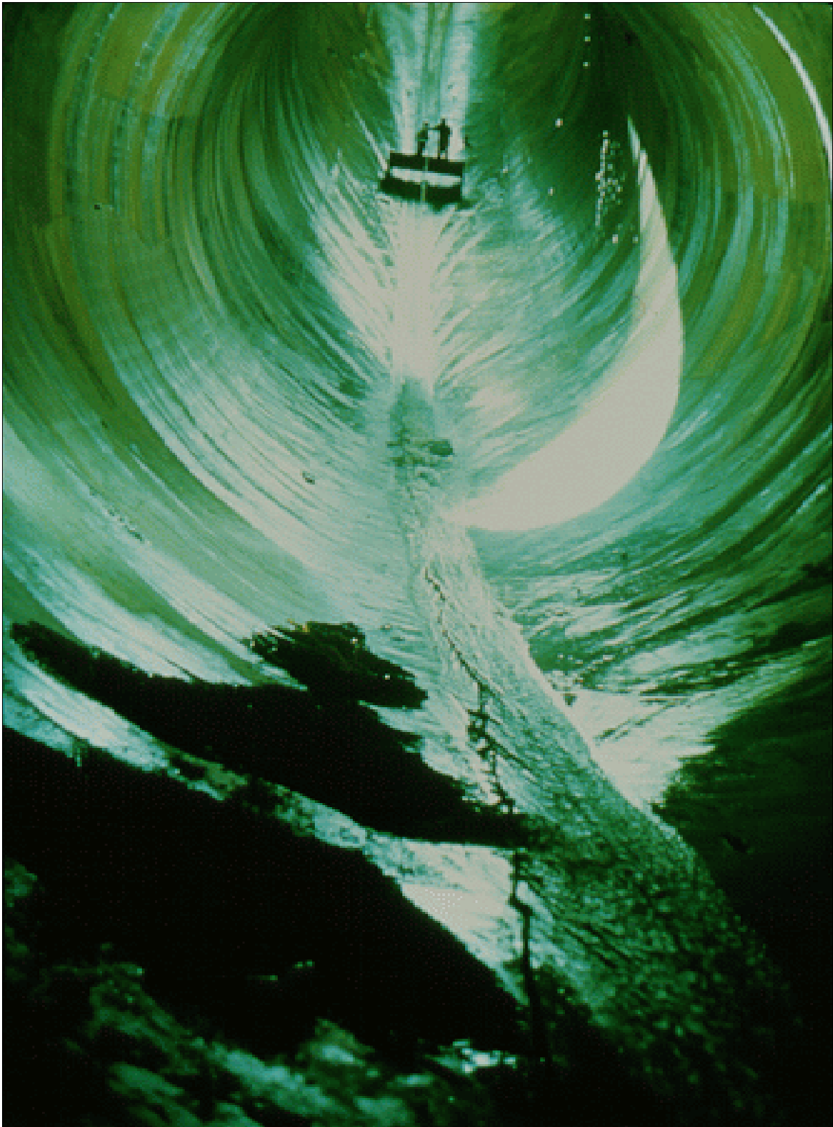
Figure 27.—Typical Christmas tree pattern of progressive cavitation damage.
