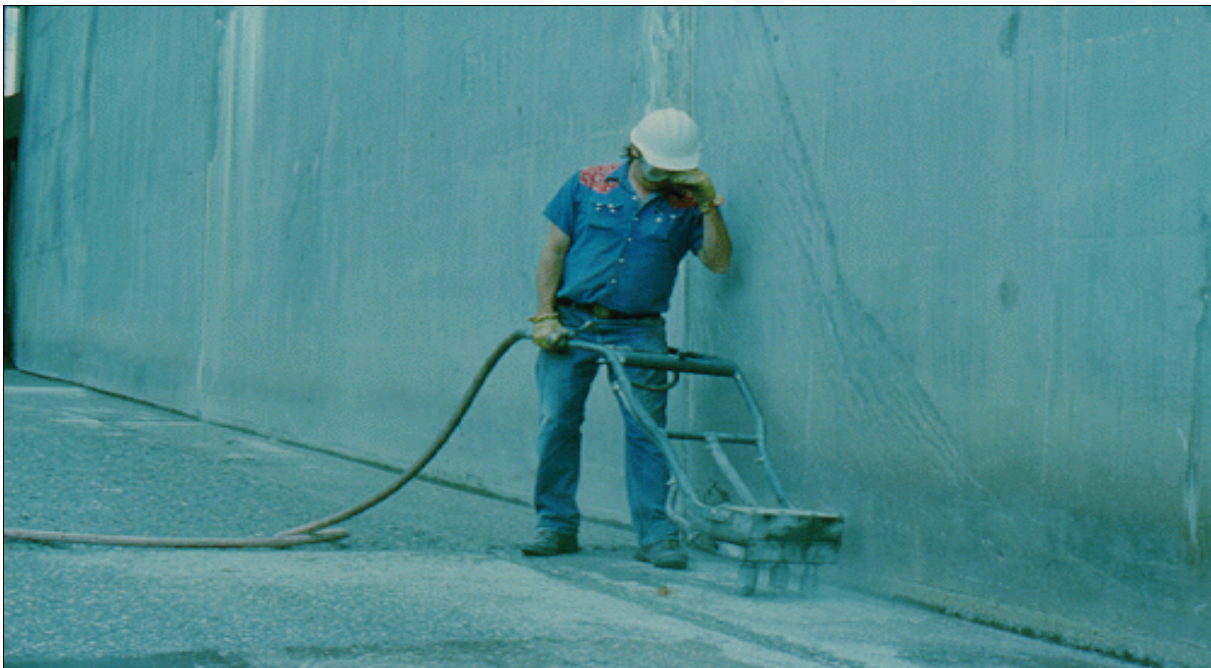
Figure 11.—Scrabbler equipment used to remove shallow concrete deterioration.
