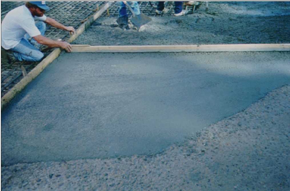
Figure 69.—This workman is hand screeding a small silica fume concrete repair.
