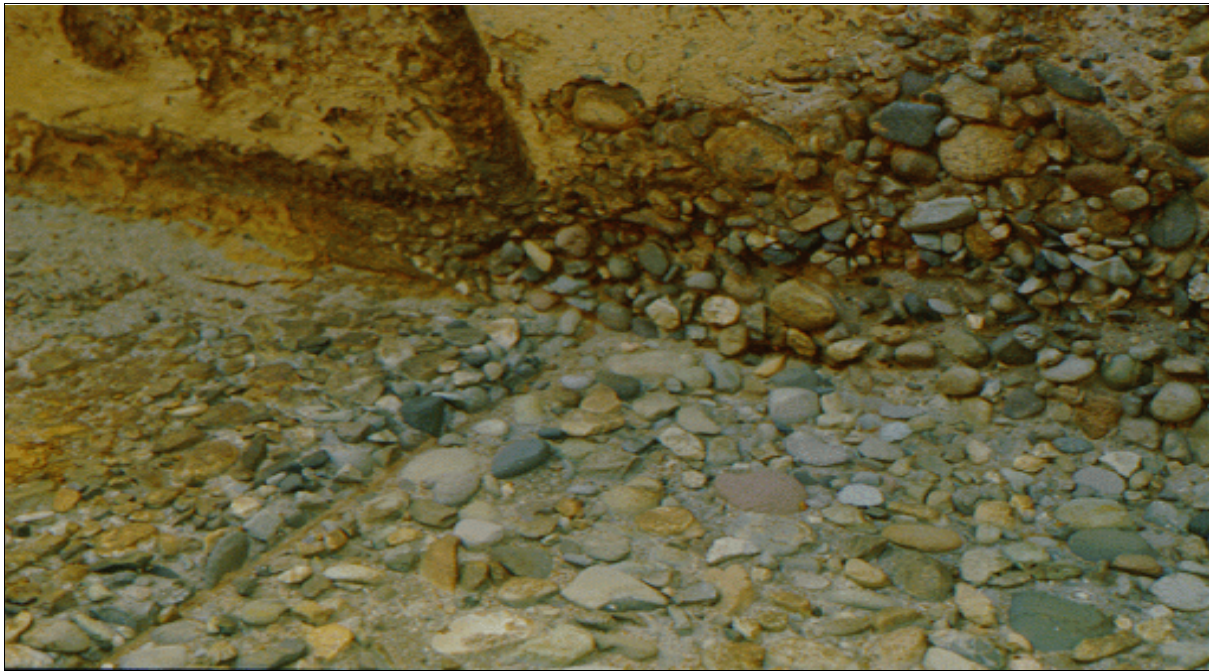
Figure 30.—Concrete deterioration caused by acidic water.
