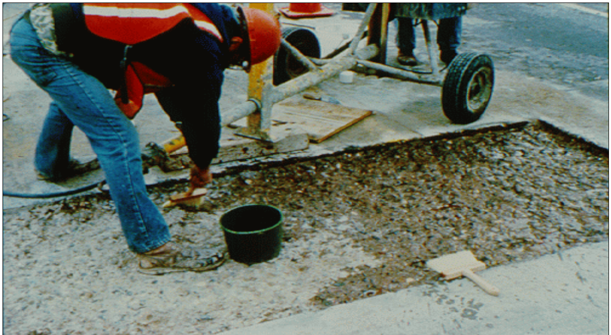
Figure 15.—Preparation of a shallow defect on a highway bridge deck.
