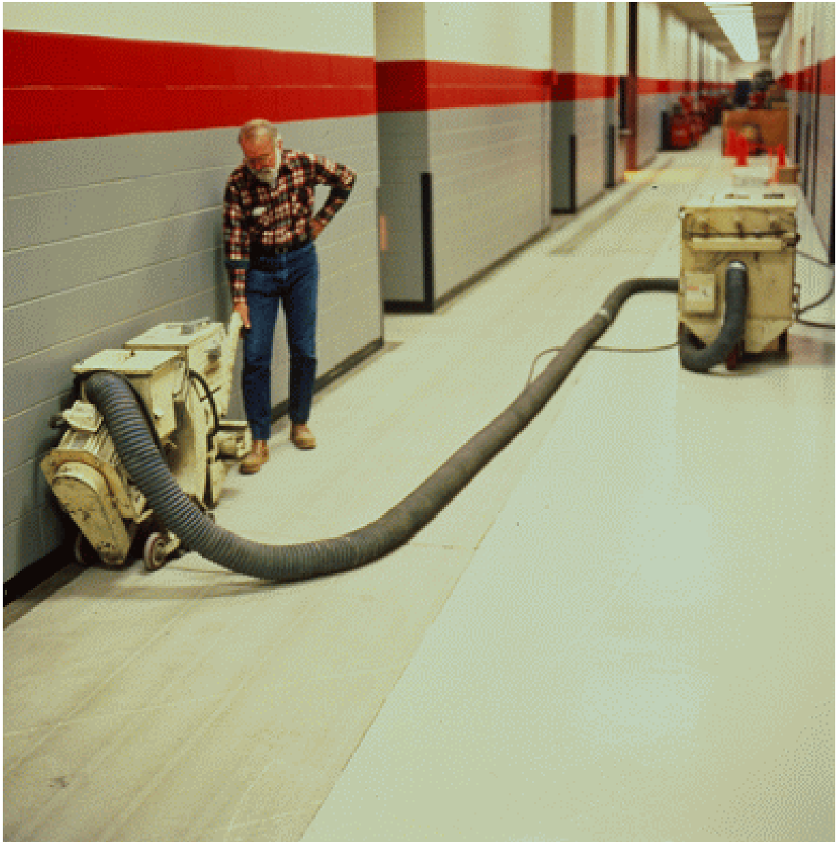
Figure 10 – Shot blasting equipment used to remove shallow concrete deterioration
