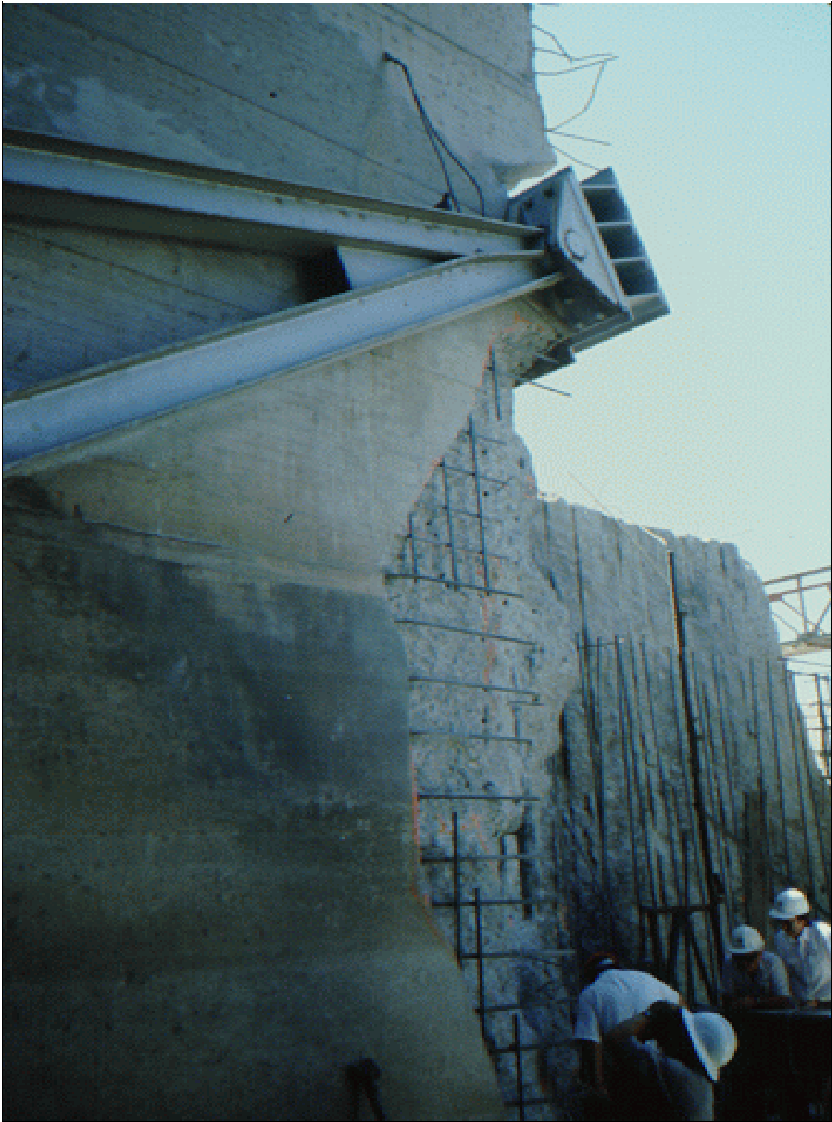
Figure 47.—Preparation of a wall for placement of replacement concrete repairs.
