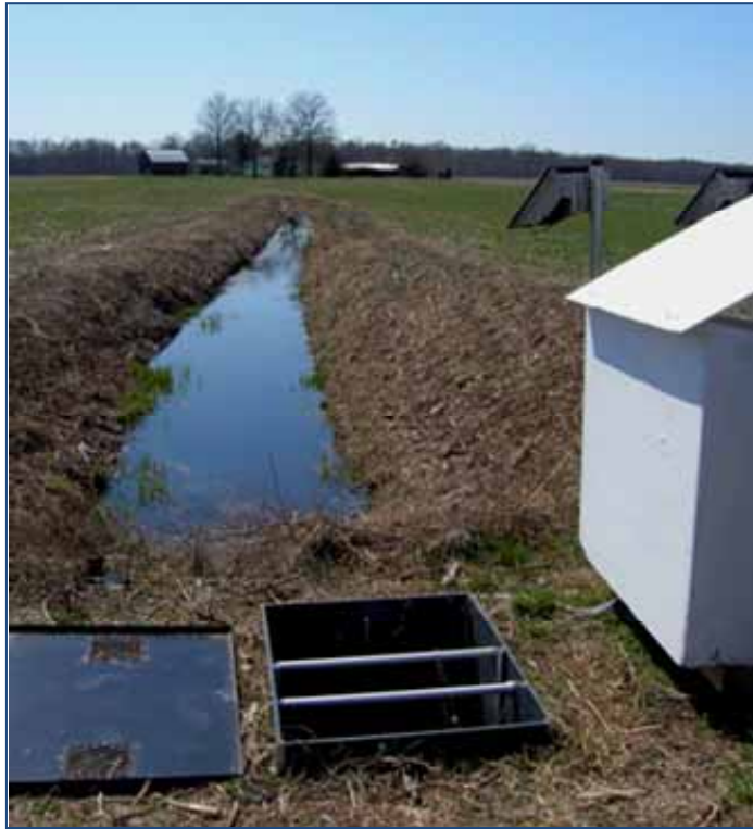
Figure 11. Controlled drainage structure and ditch equipped with flow monitoring and sampling equipment (above). Top view of controlled drainage structure. Boards can be added and removed to adjust water levels (right).
