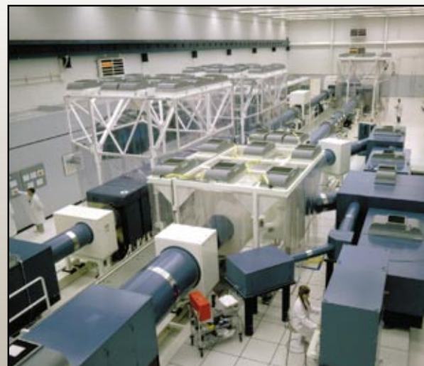
The Beamlet Demonstration Project has been ongoing since 1990 to develop, test, and refine NIF's laser design and hardware.
