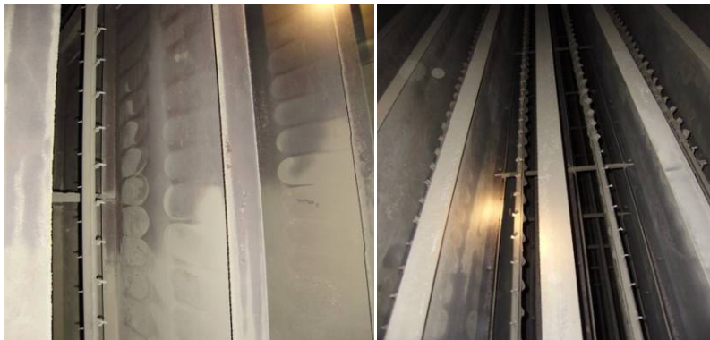
Figure 2.3.1-3 Unit 3's and 4's PPTR plates and electrodes
