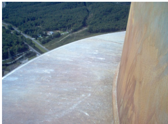
Figure 2.2-3. This picture was taken at the top of S1. Again, white material deposited here is presumed to be the flake material that exited the stack on September 10 th and 18 th .
