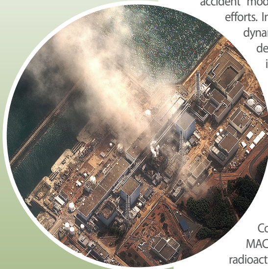
Damaged reactor buildings from the Fukushima Daiichi Nuclear Power Plant
