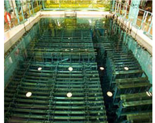
Spent fuel pool assembly similar to those modeled by MELCOR
