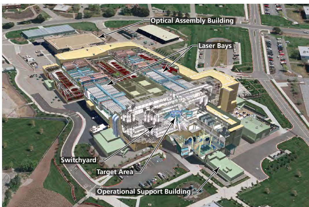
Figure 1-1: NIF aerial view, showing the two laser bays, switchyard, target chamber area, Operational Support Building, and Optics Assembly Building.
