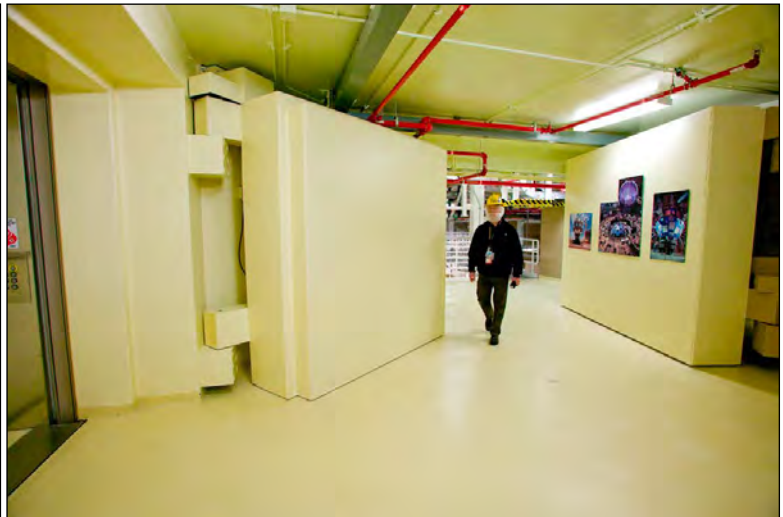
Figure 4-2 (left): High-resolution models of the NIF facility are used to perform both prompt and post-shot calculations for estimating radiation levels in the facility. Figure 4-3 (right): Completion of shield doors and other shielding elements helped enable NIF to ramp up shot neutron yields. Shown above is one of the 44 shield doors installed throughout the NIF.
