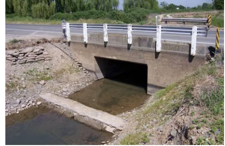
Colusa Highway Bridge
