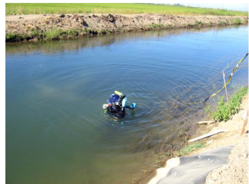
FIGURE A-4 Diver Installing Flow Meter
