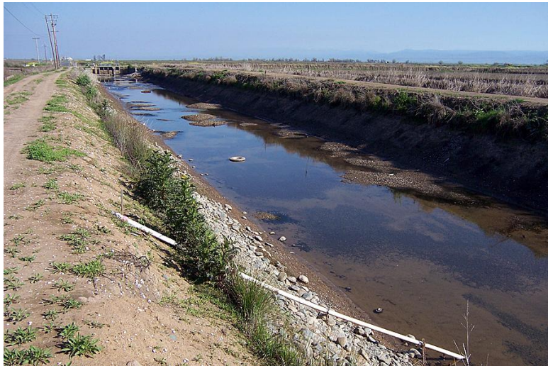
FIGURE 3-1 Typical Water Level Sensor Installation during Annual System Shutdown
