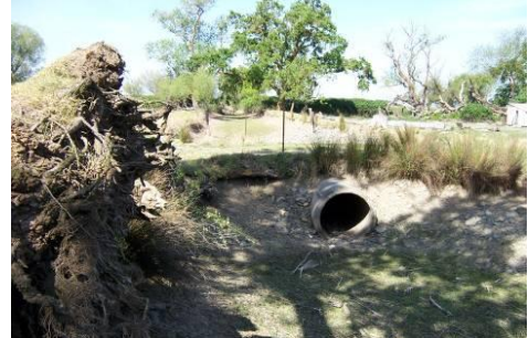
Culvert Upstream of Bonslett Driveway
