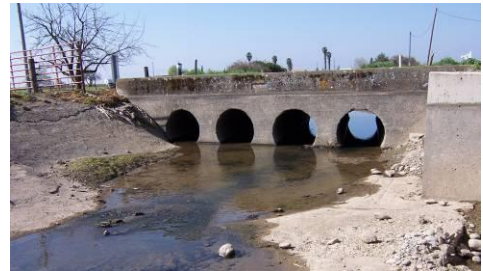
Farris Road Bridge
