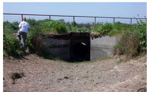
Concrete Pipe Culvert #1163
