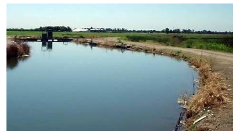
Typical Existing Reach of the Belding Lateral
