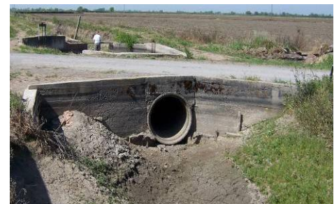
Bonslett Driveway Culvert and Crossing #1199
