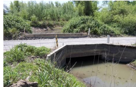
Evans Reimer Road Bridge
