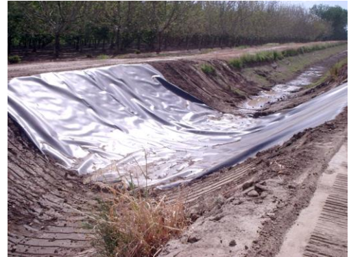
FIGURE A-2 Canal Lining
